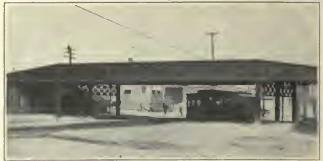
FIG. 278. TRACK ELEVATION. Double track plate-girder span on the Chicago, Milwaukee & St. Paul Railway at Healy Station.
